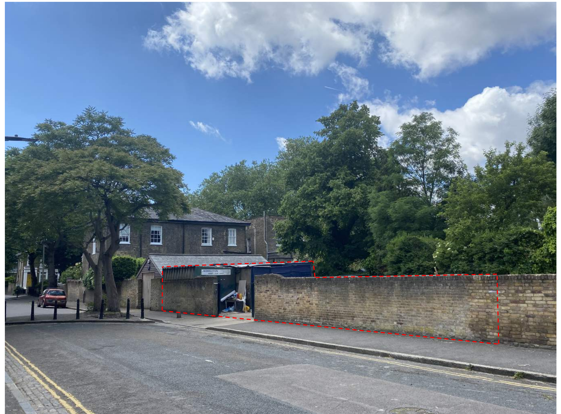
Site as seen from the northern end of Albion Square
