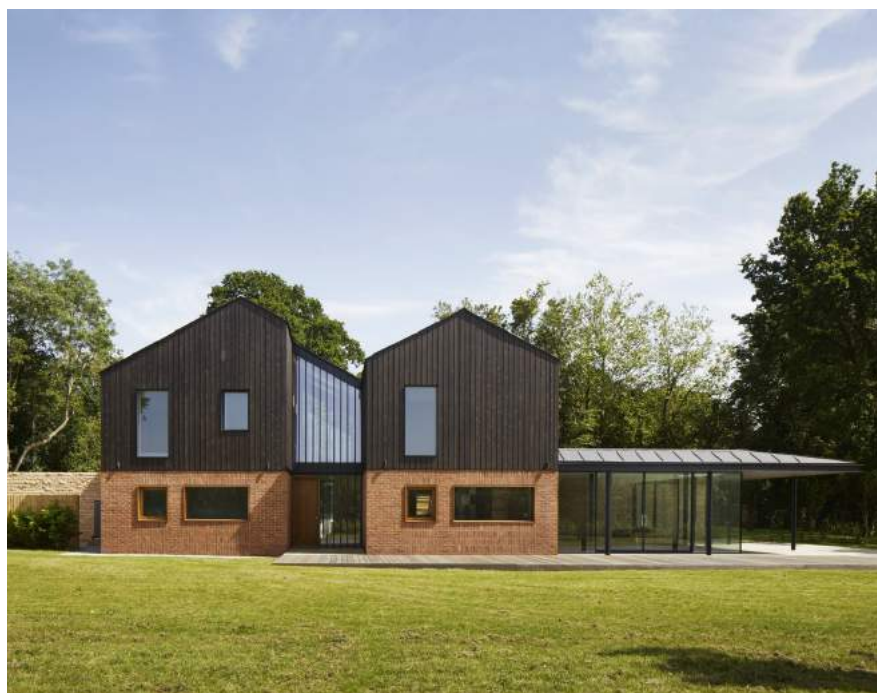
Split House, Windsor, Berkshire
